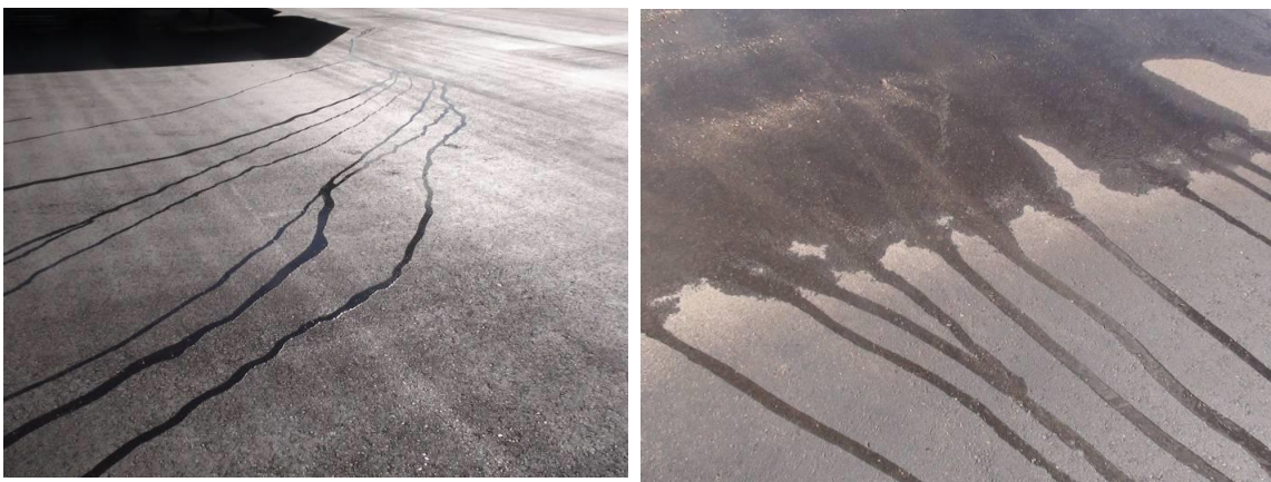
Figure 5. Fast removal of runoff water on asphalt pavement surface treated with RePlay® (BPS 2014).
